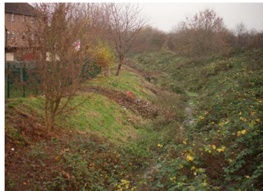
New fencing and cleared embankment November 2006
